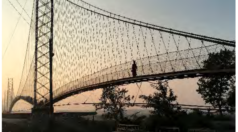
Dodhara Chandari Suspension Bridge, Kanchanpur, Province 7 © ICTJ
